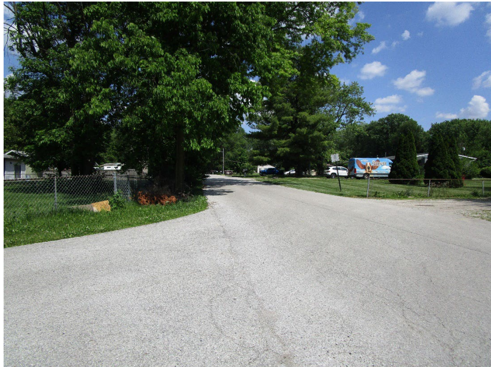
View looking east along East Sumner Avenue
