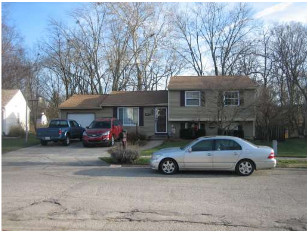
Adjacent dwelling to the east, looking south
