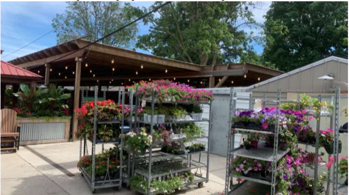
Full view of the proposed greenhouse location and garage to be demolished.
