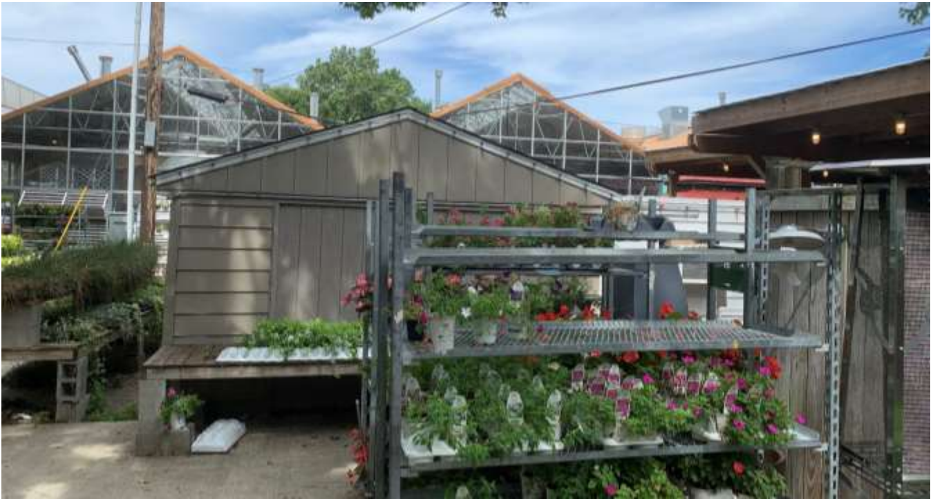
Photo of the existing detached garage to be demolished on the west side of the existing fence line.
