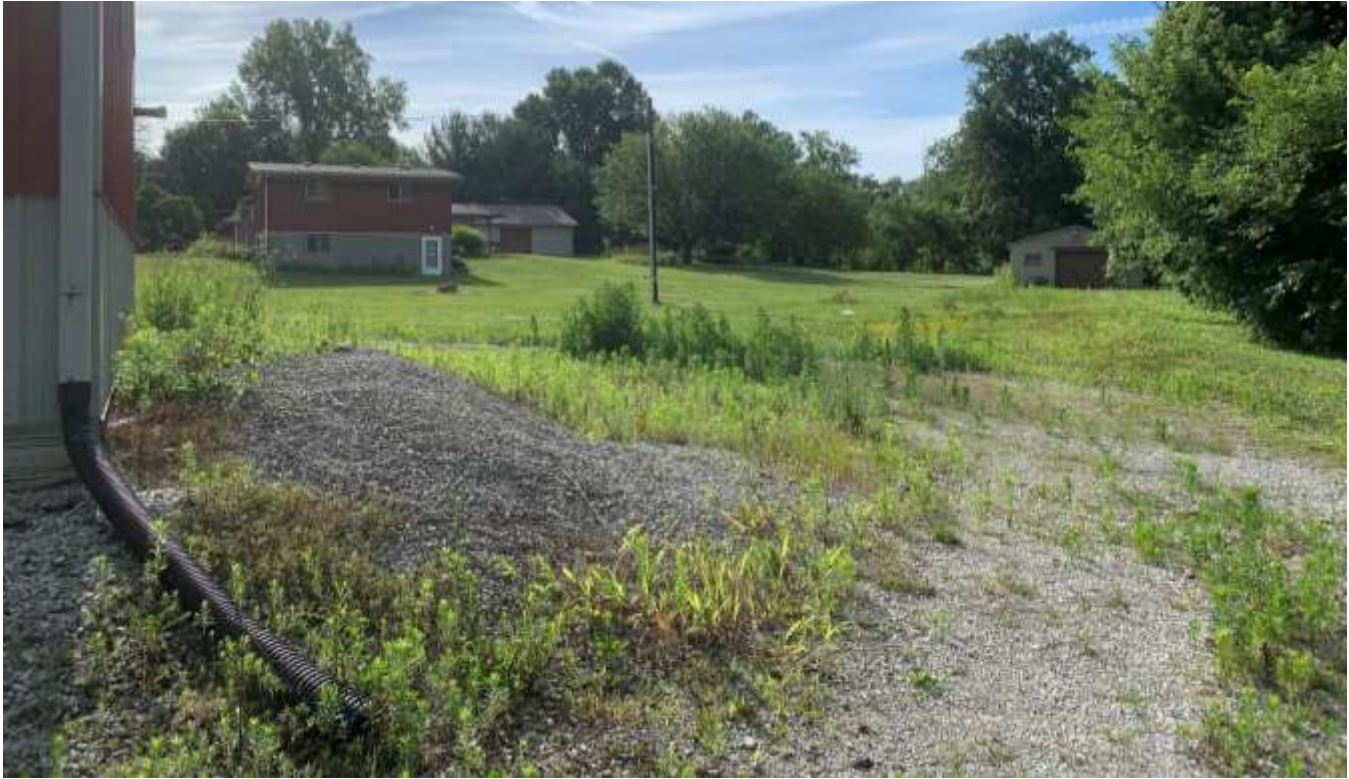
Photo of the stream protection corridor to the right where the two existing garages are located.
