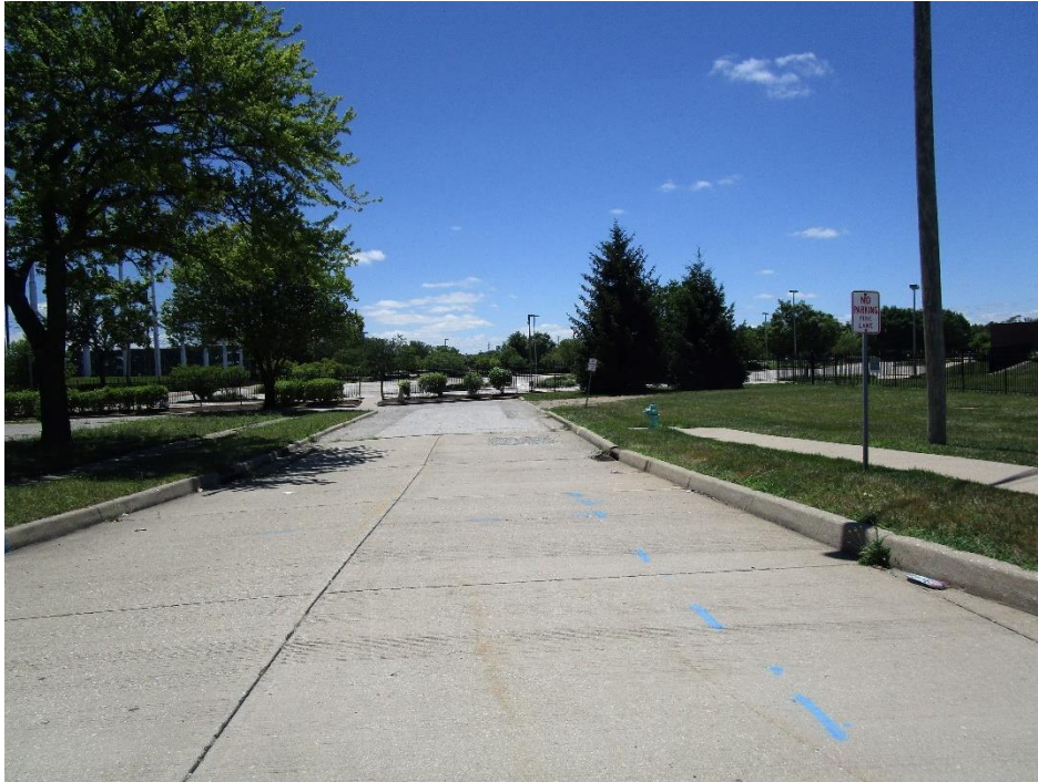
View looking south along Bridge Street
