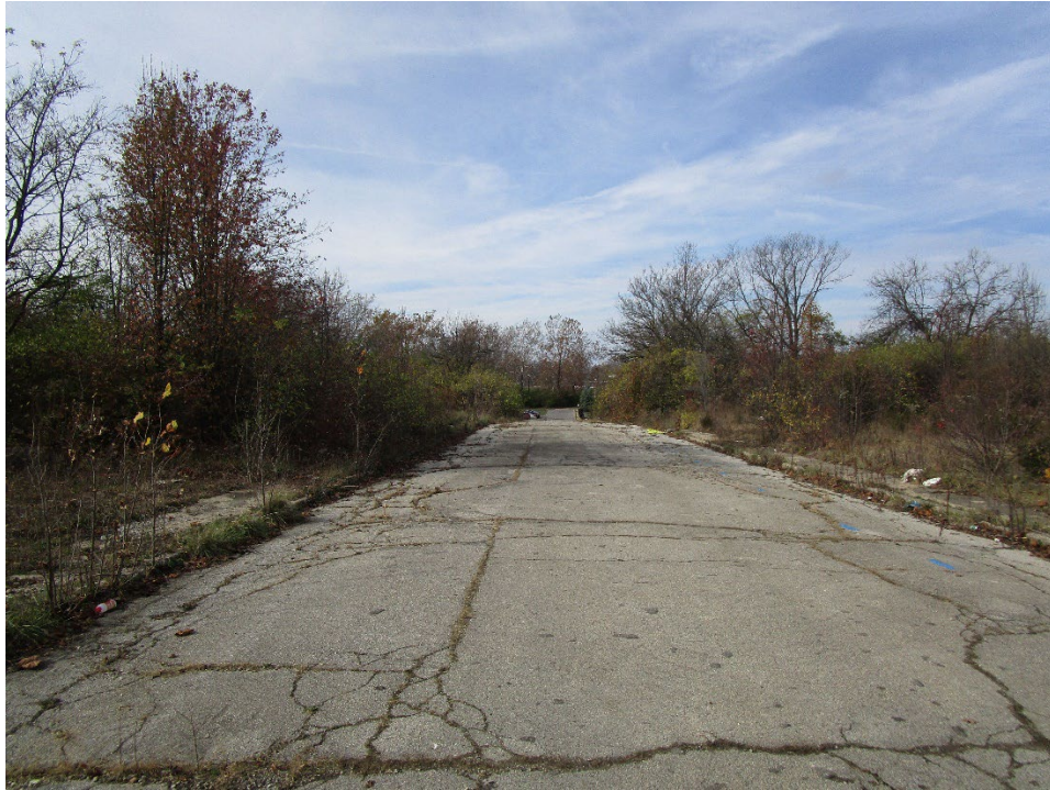
View looking east along Adams Street
