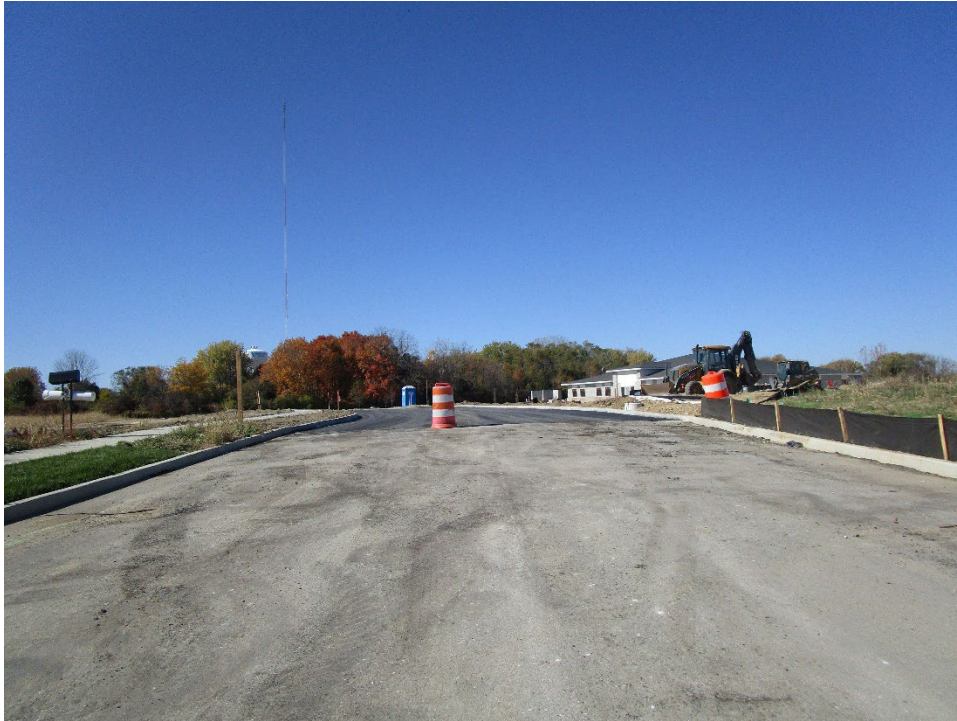
View looking west along private drive
