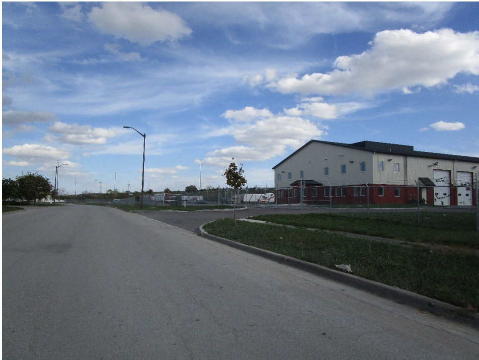
View of site looking southwest across Enterprise Park Place
