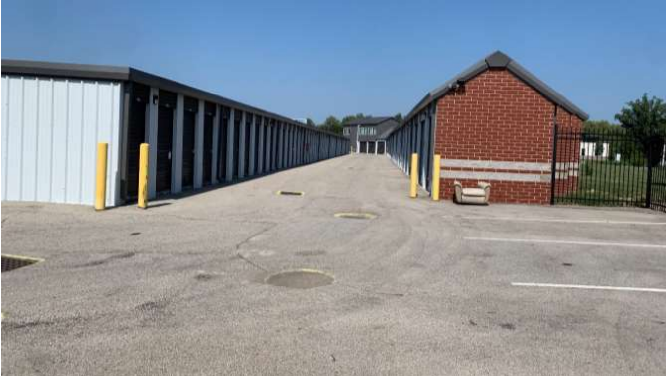
Photo of the storage facility looking northeast.
