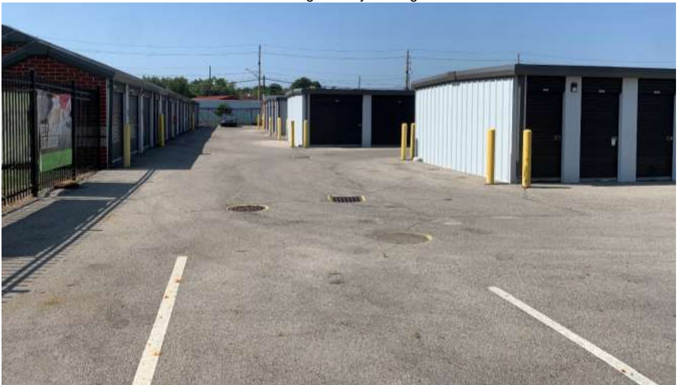
Photo of the storage facility looking northwest from Binford Boulevard.
