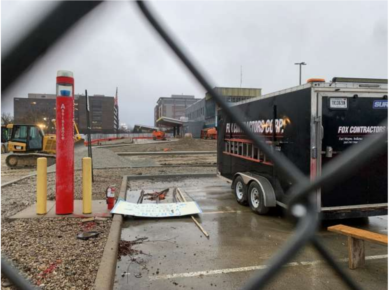
Location of the proposed freestanding sign looking south.
