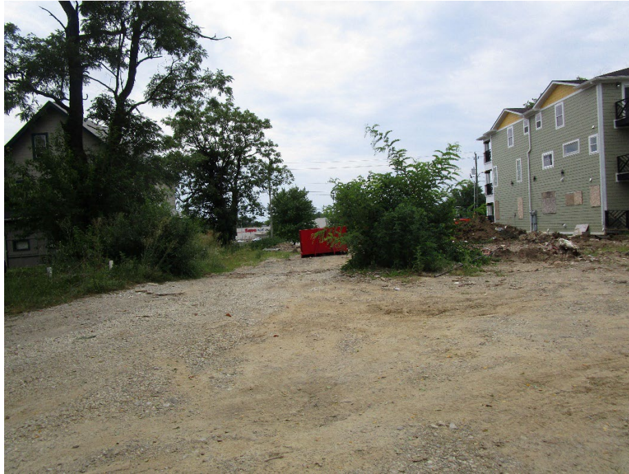
View of site looking south from the east / west alley to the north
