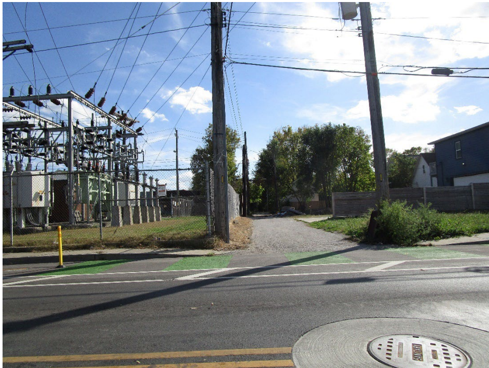
View of abutting north / south alley to the east of site
