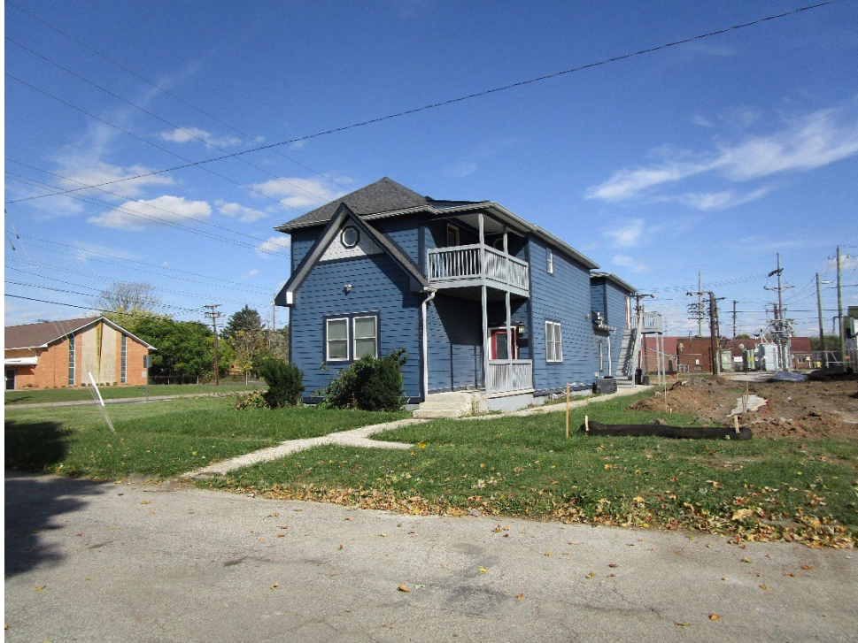
View of site looking northeast across Columbia Avenue
