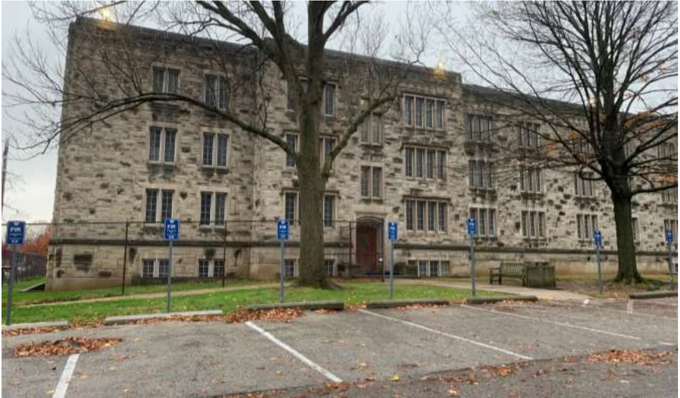
Photo of the eastern building façade of the dormitory on site.
