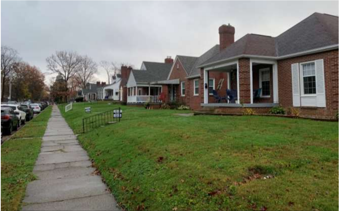
Photo of single-family dwellings south of the site.
