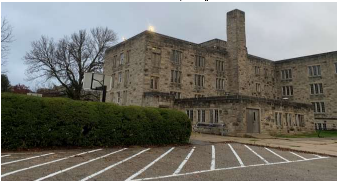
Photo of the dormitory looking northeast.
