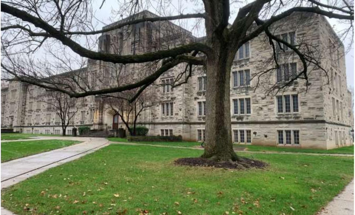
Photo of the northern building façade of the dormitory on site.
