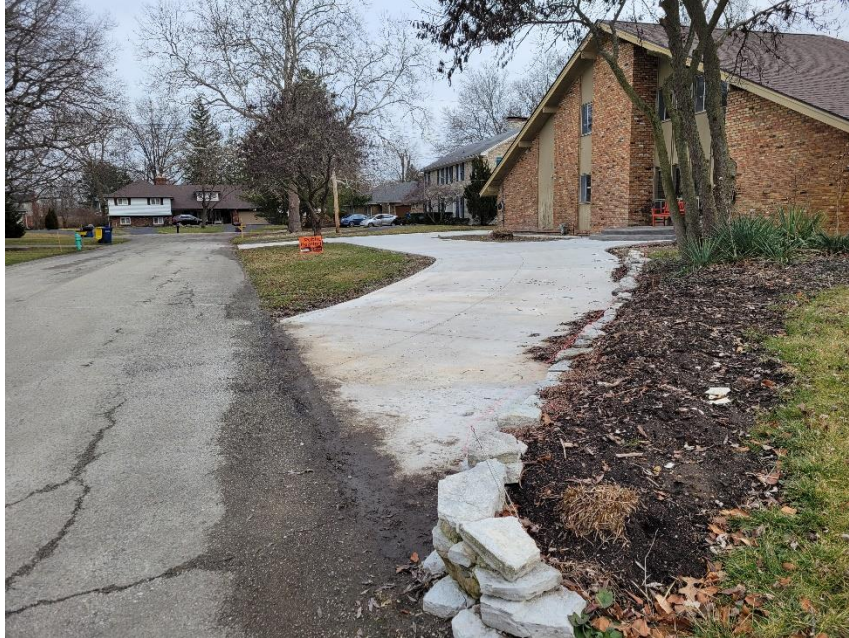
Photo 5: Existing Driveway/Parking Area in Front Yard (North)
