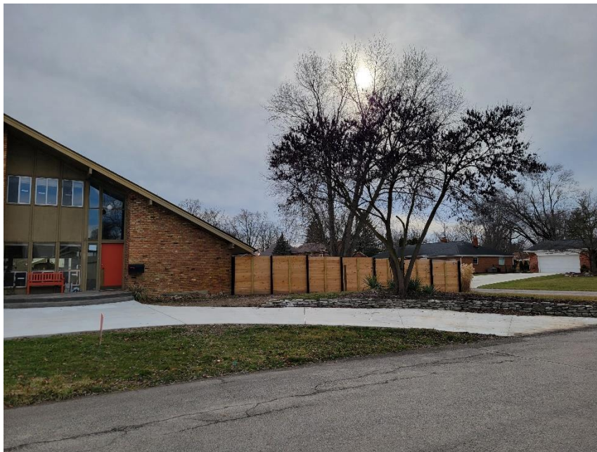
Photo 4: Fence and Property from Front Yard (North)
