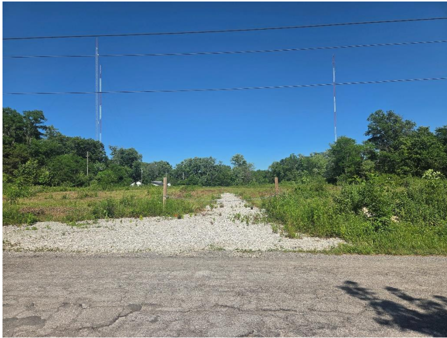
Photo 3: Extension of 78 th Street Viewed from Walnut to West
