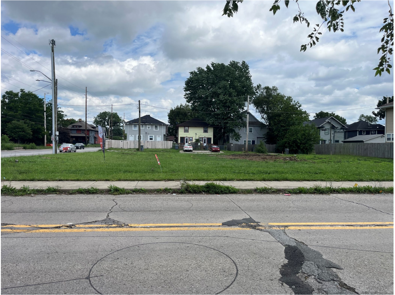
Photo 1: View of subject site as seen from Ruckle Street
