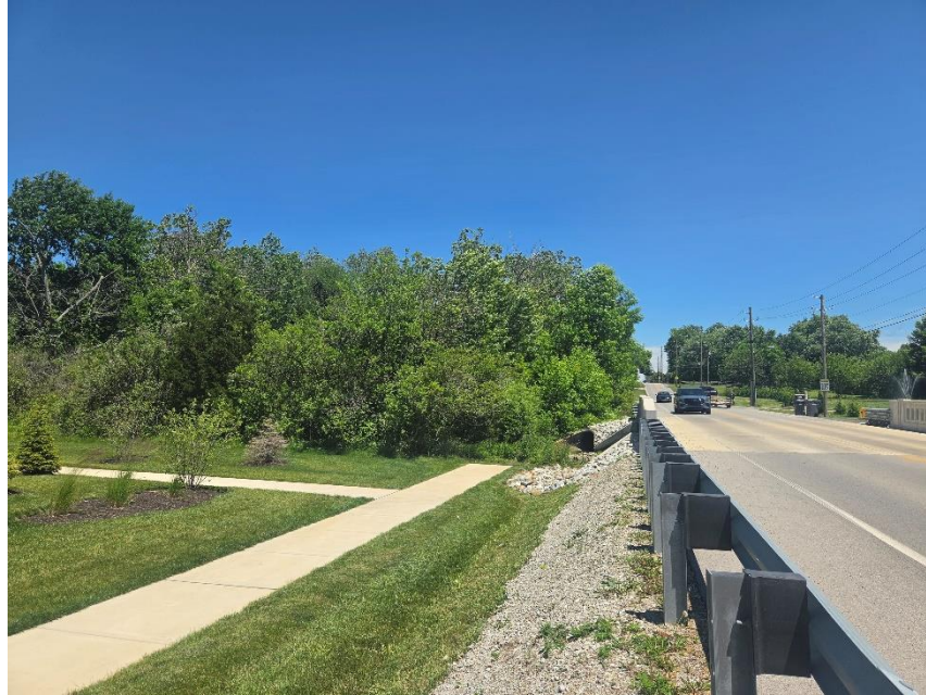
Photo 3: Horn Creek Bridge Viewed from West
