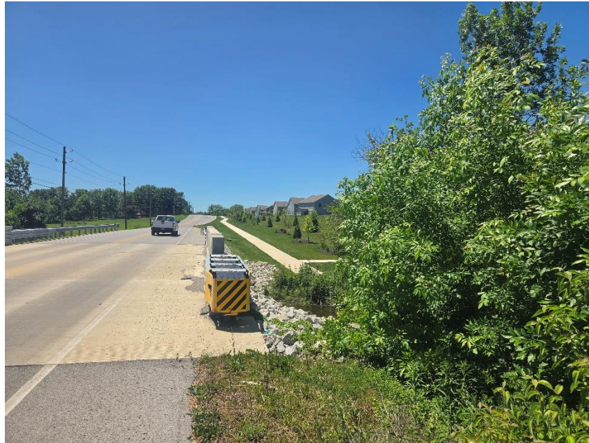
Photo 5: Horn Creek Bridge Viewed from East
