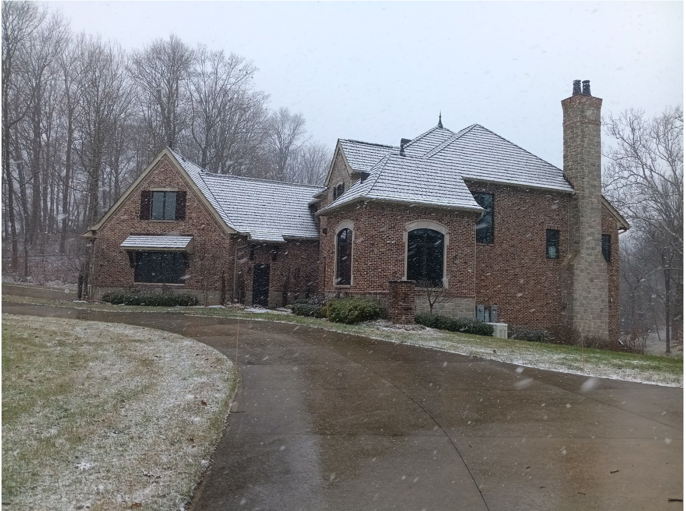
Exhibit 6: The primary structure at 8654 West 86 th Street.
