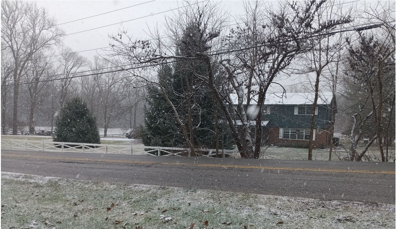
Exhibit 12: The home across the street from 8654 West 86 th Street with their existing within compliance fence.
