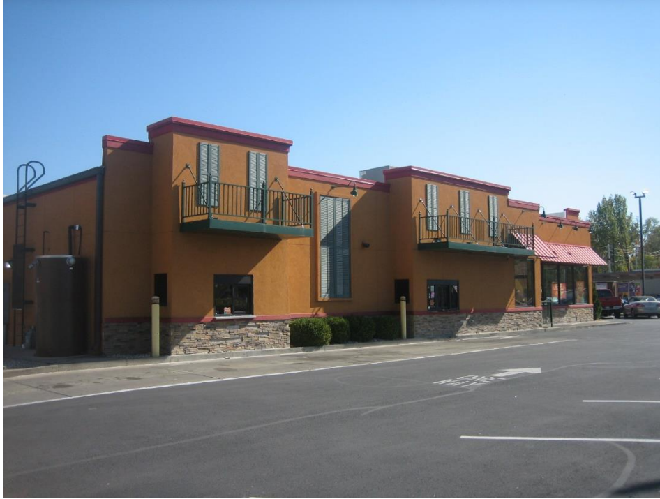
Subject site drive thru stacking spaces in front yard of North Keystone Avenue, looking southeast.
