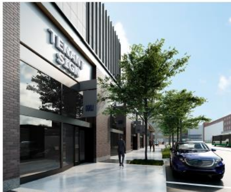
View from sidewalk along N. Capitol Avenue.
