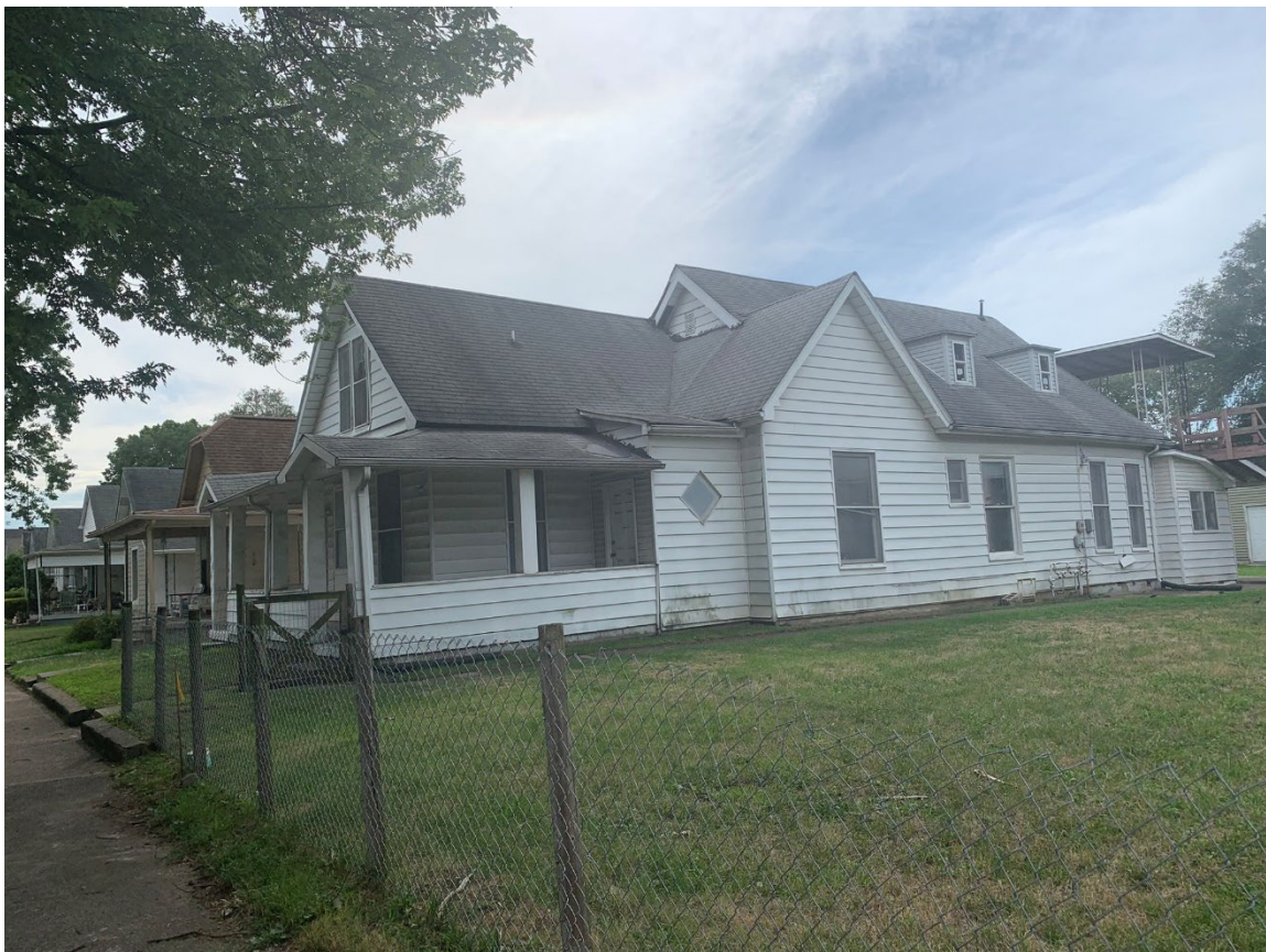
Views of neighboring structures
