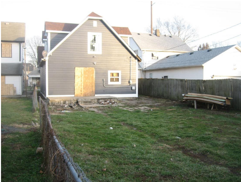
Subject site rear yard, looking southeast
