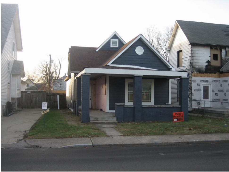
Subject site, looking west from Belmont Avenue.
