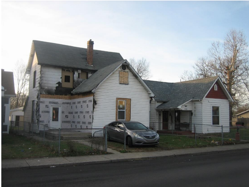
Adjacent single-family dwellings to the north, looking northwest
