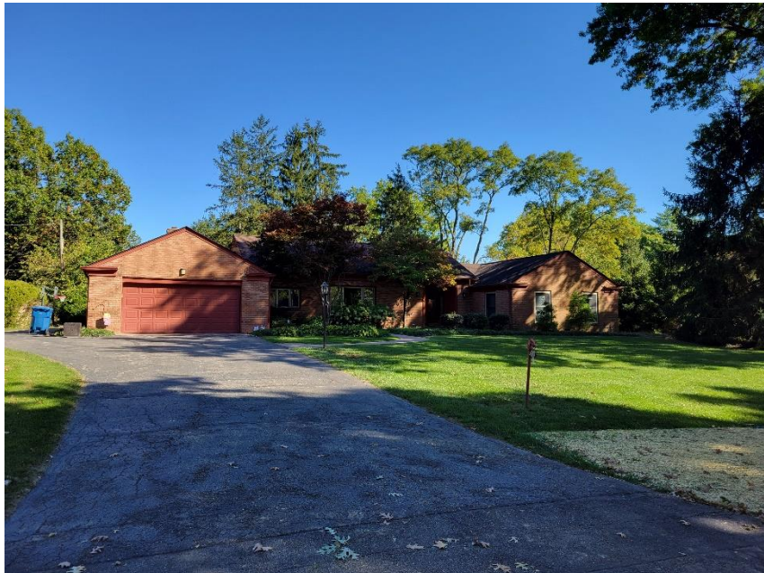
Photo 2: Subject Site from West
