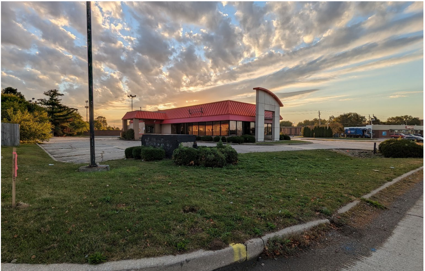
Photo of the Subject Property, view from north
