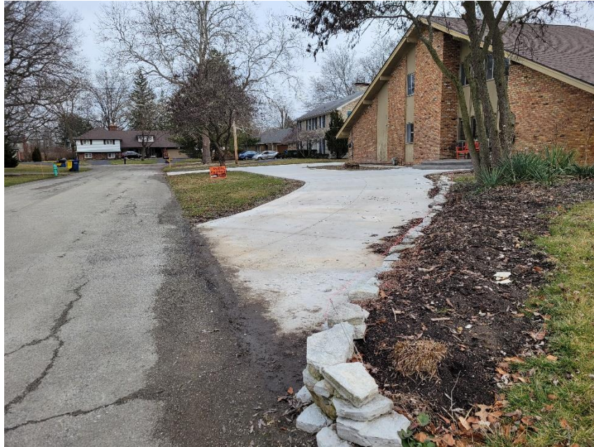
Photo 5: Existing Driveway/Parking Area in Front Yard (North)
