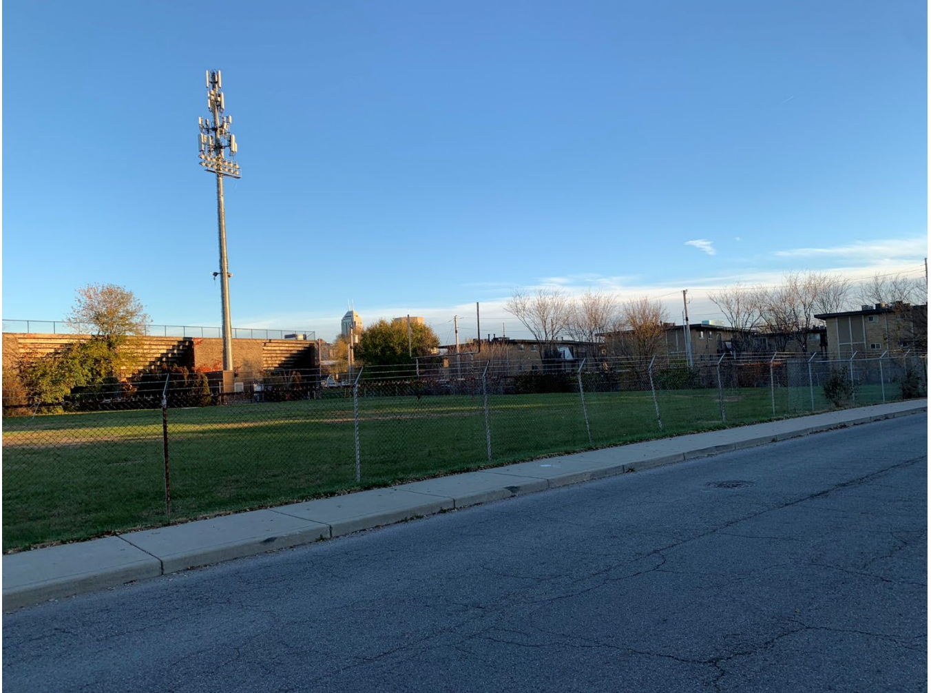
Existing wireless communications facility, from Brooks Street
