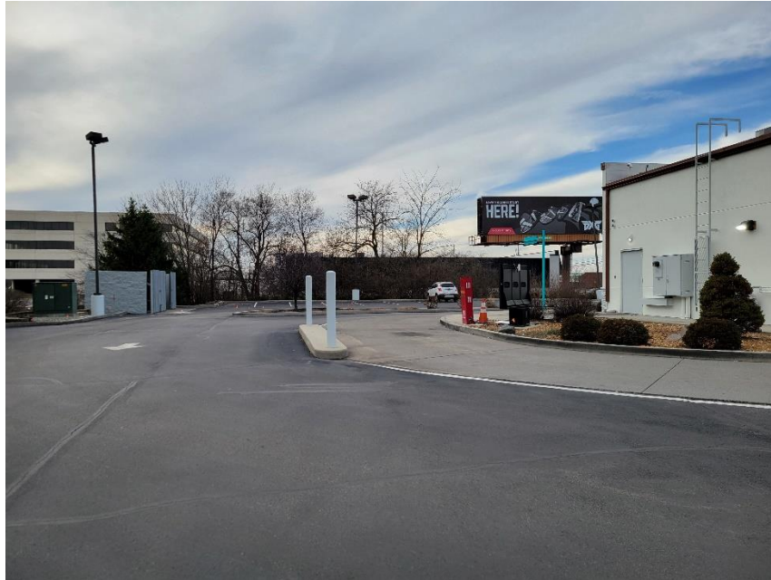
Photo 5: Existing Drive-Thru Menu Board from East
