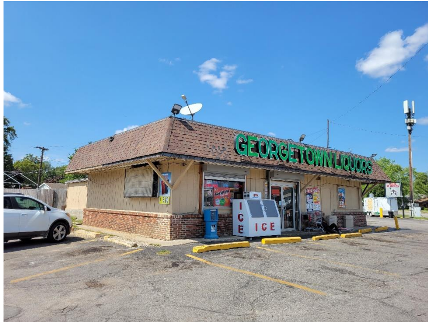
Photo 1: Subject Site Viewed from Southwest
