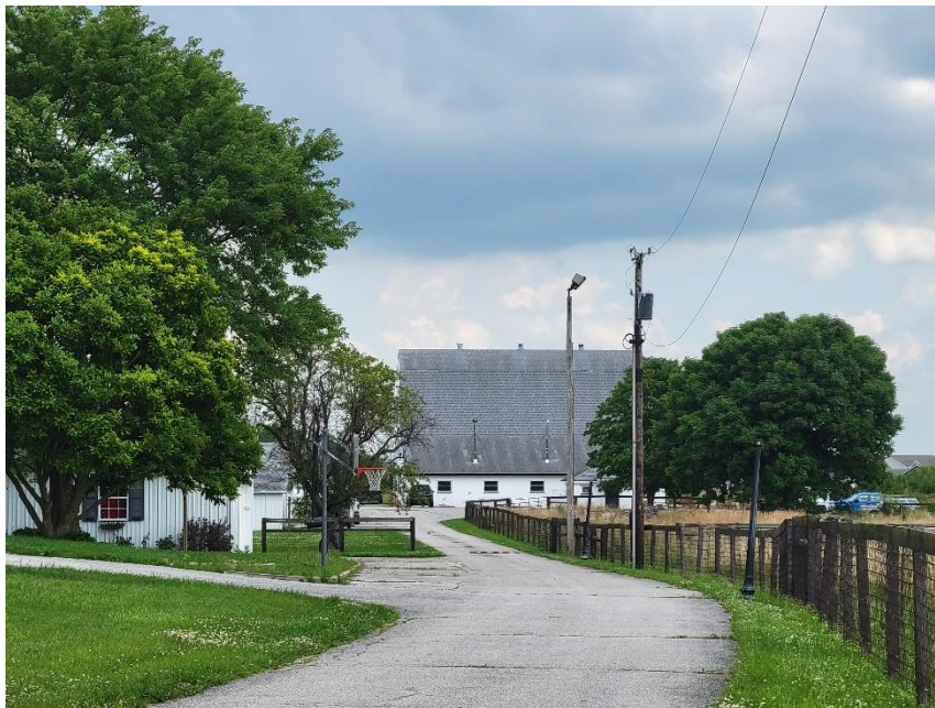
Photo 2: Existing Rear Buildings viewed from West
