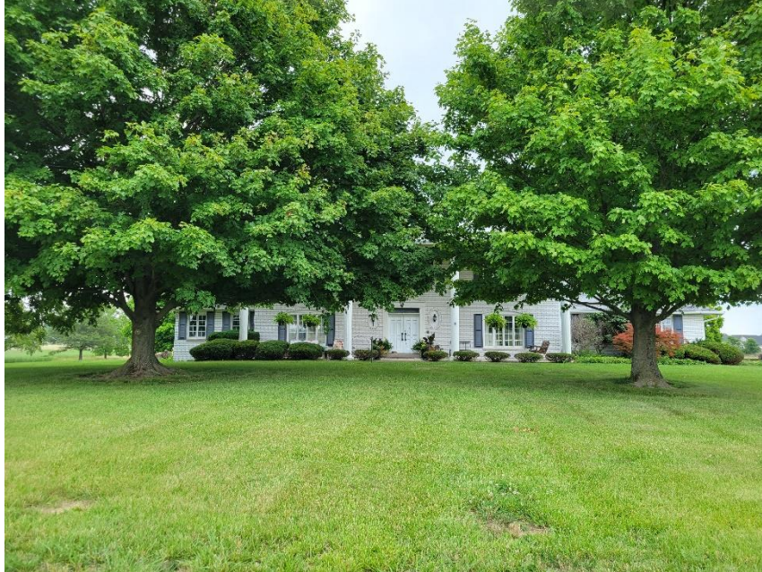
Photo 1: Existing House viewed from West
