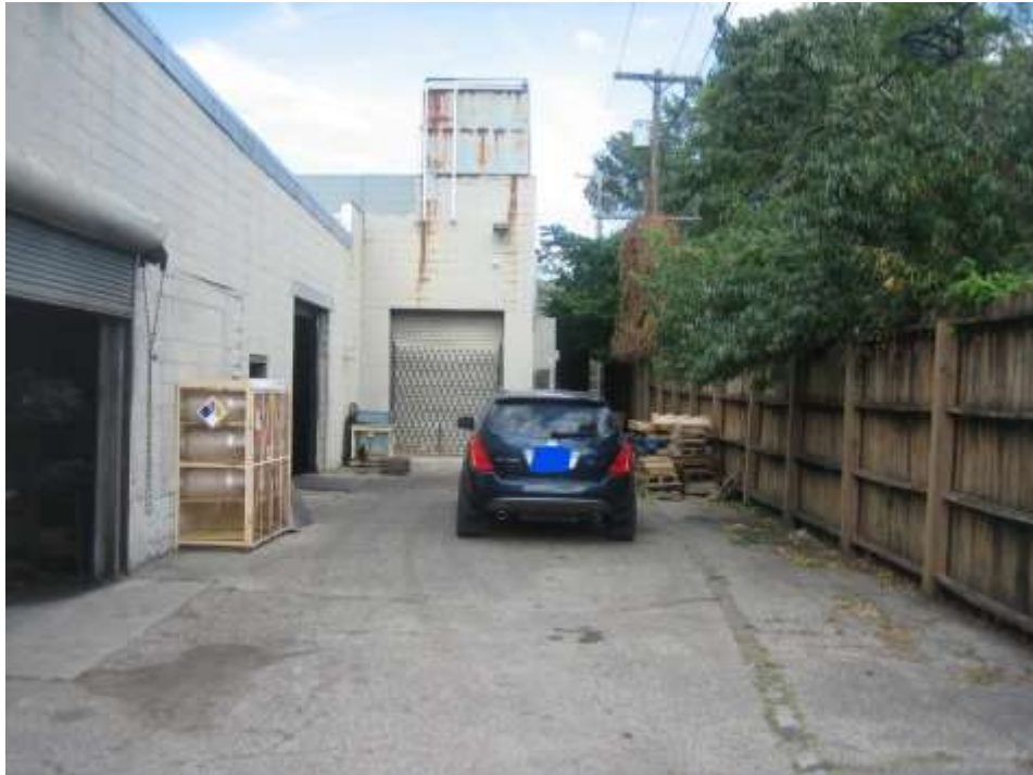
Subject site 2343 Massachusetts Avenue rear of building, looking northeast
