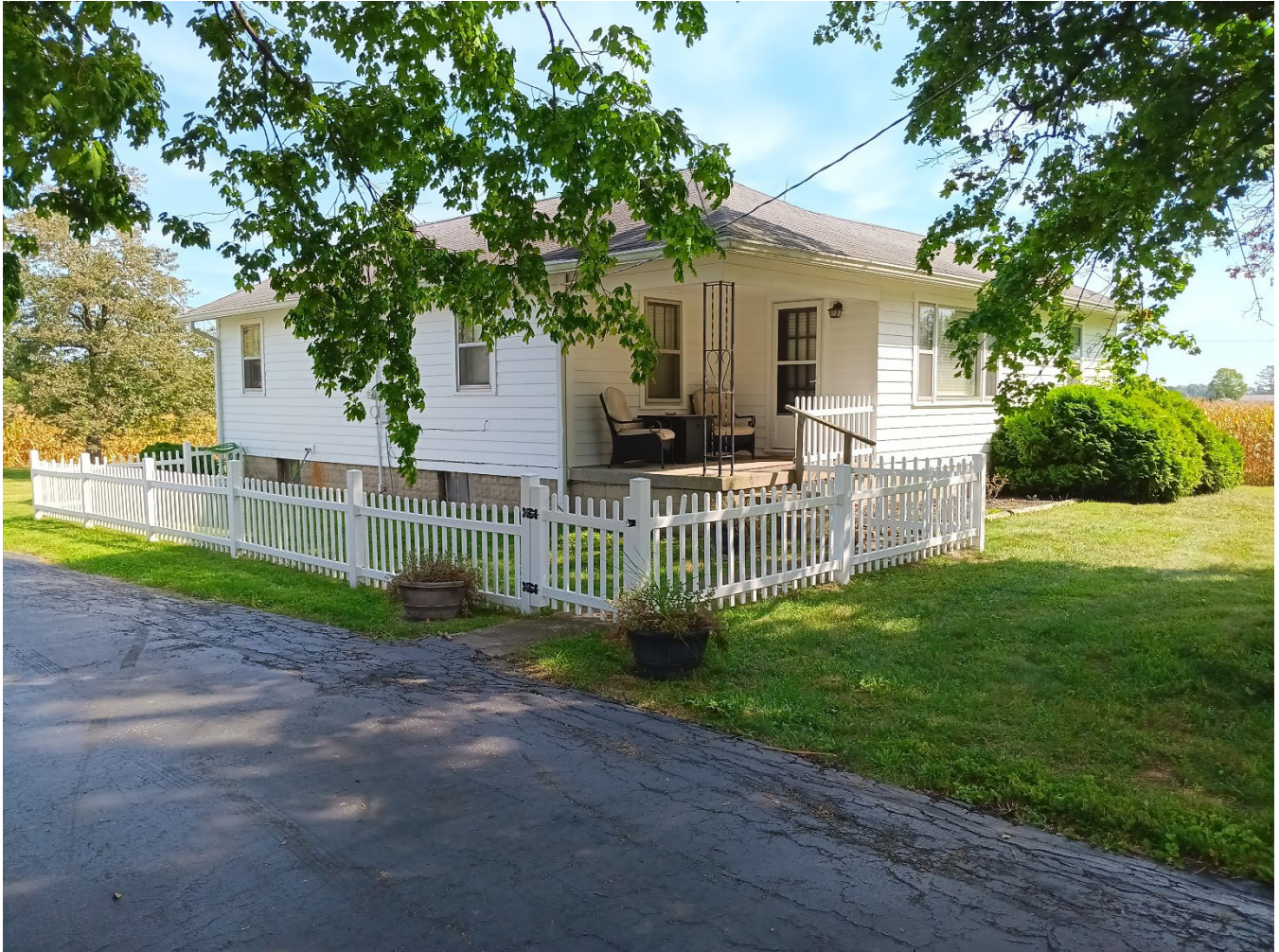
Exhibit 4: Existing home on 9540 Maze Road.
