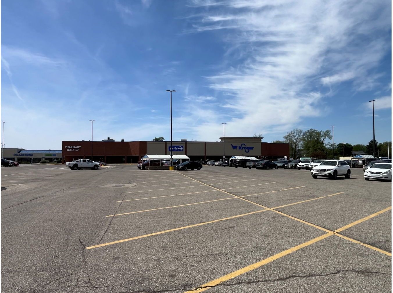
Photo 5: Integrated center where gas station sits
