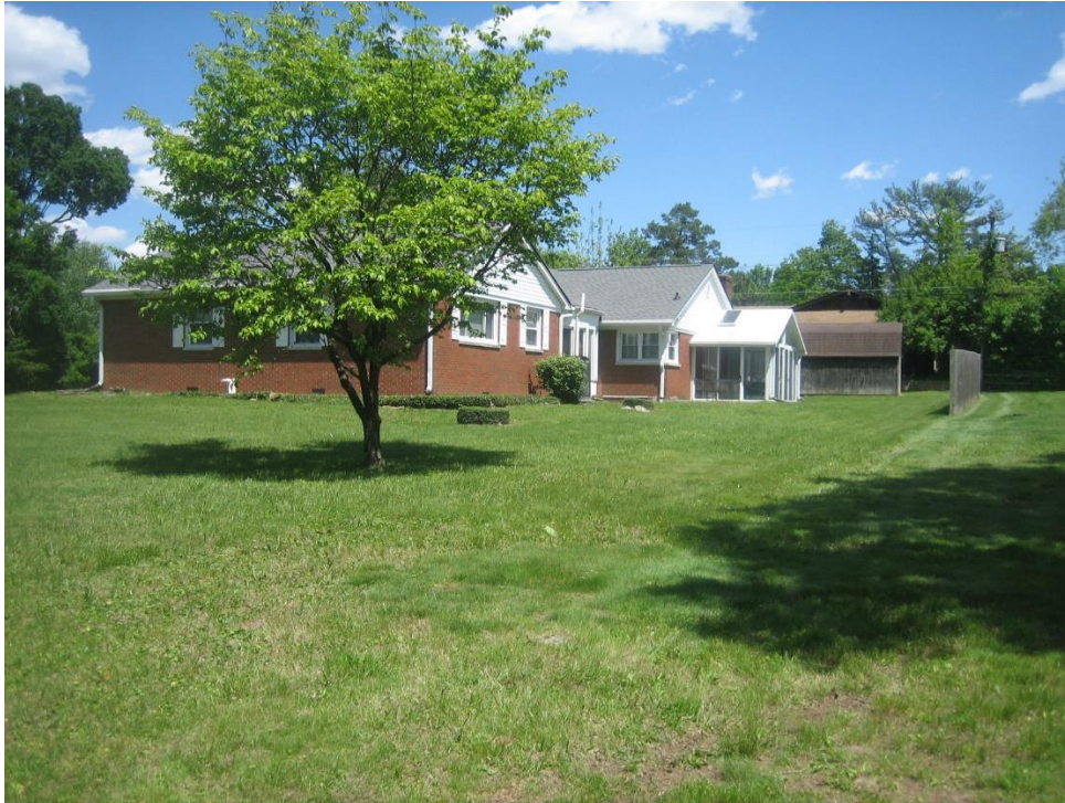
Adjacent dwelling to the north, looking northeast
