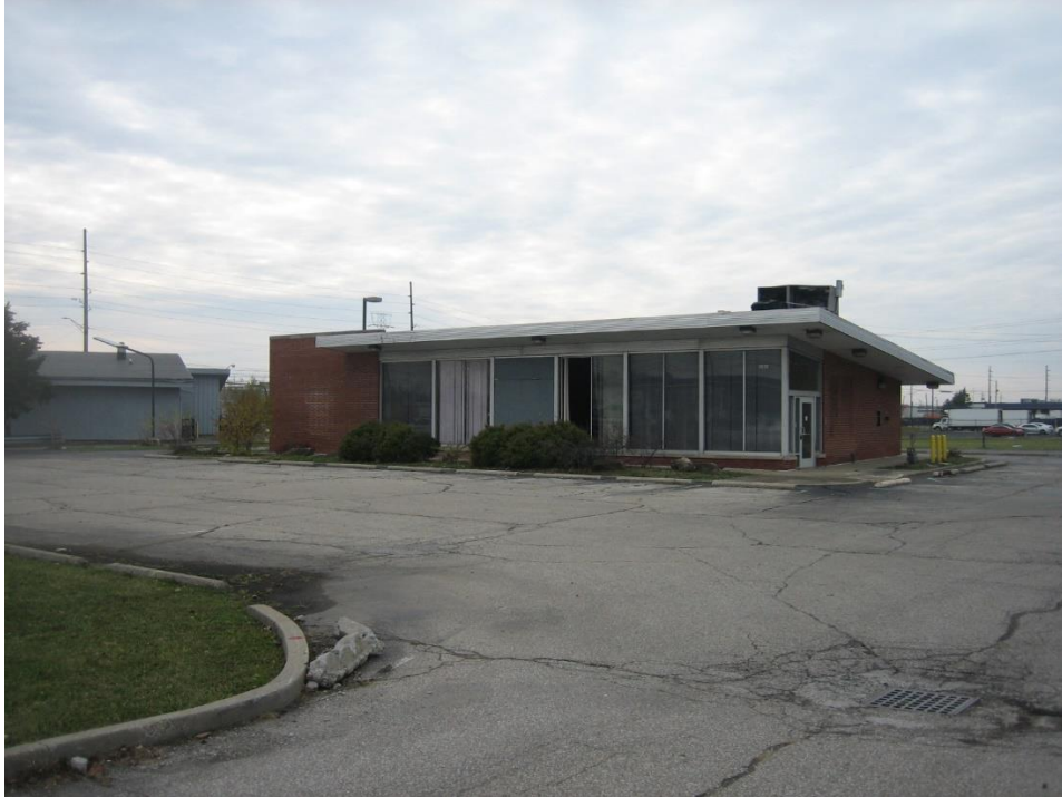
Subject site existing building, looking west.
