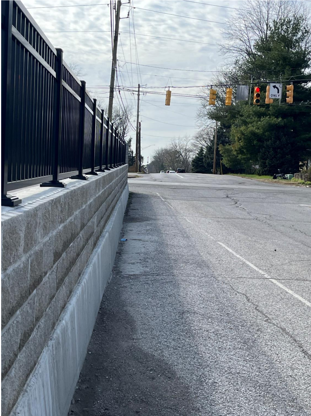
Photo 4: Fence/wall along Sumner near intersection with South Meridian
