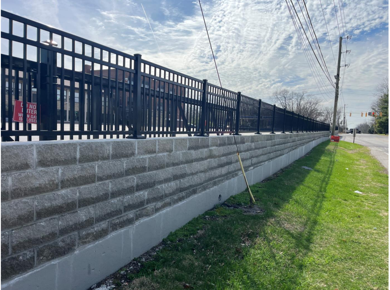
Photo 1: Fence/wall as seen from Sumner Avenue looking south
