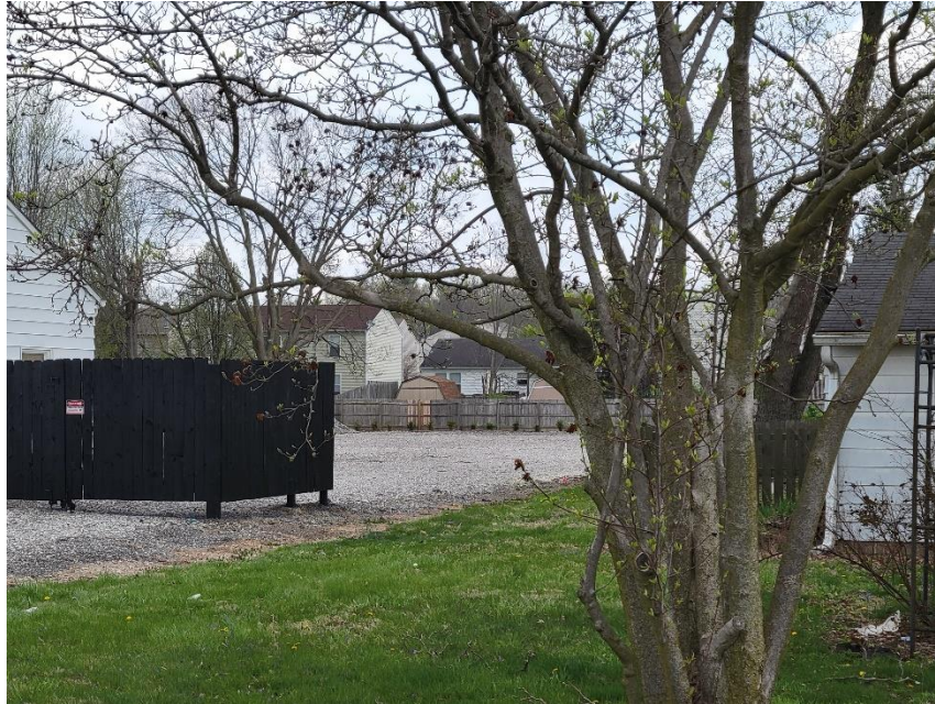
Photo 3: Rear Gravel Area Behind Fence Viewed from Southeast
