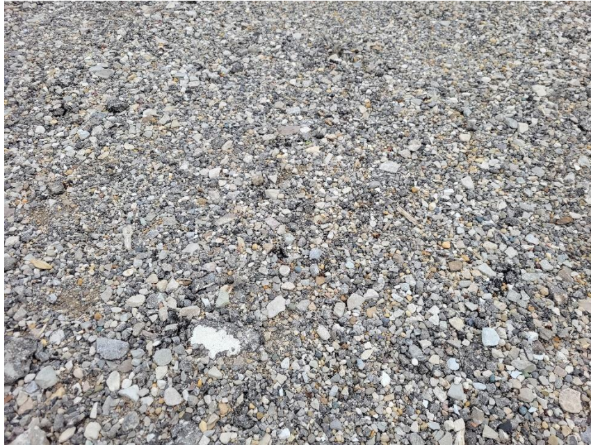
Photo 5: Surface of Parking Area
