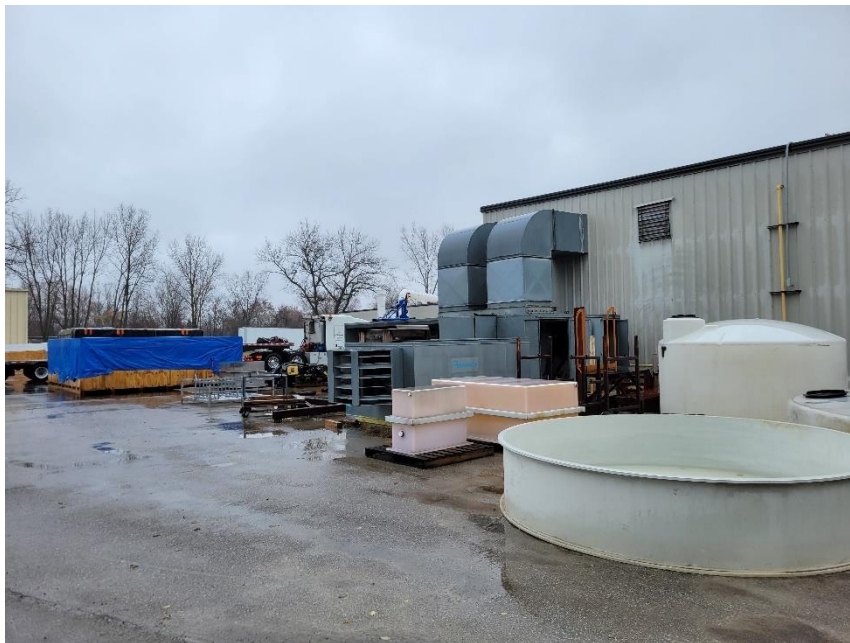
Photo 8: Southern Storage Area Viewed from Southeast
