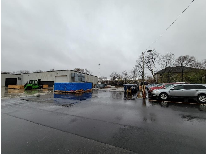
Photo 7: Southern Storage Area Viewed from Northwest
