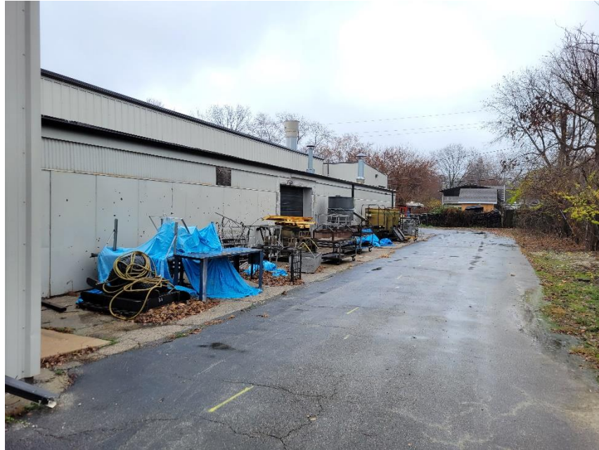
Photo 11: Portion of Primary Building (Southeast)
