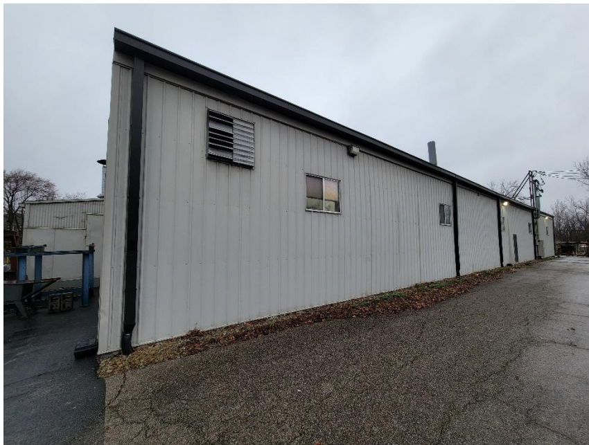
Photo 10: Primary Building Viewed from Southeast
