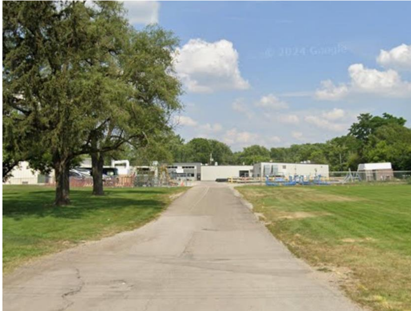
Photo 17: Subject Site Viewed from Emerson (June 2024)
