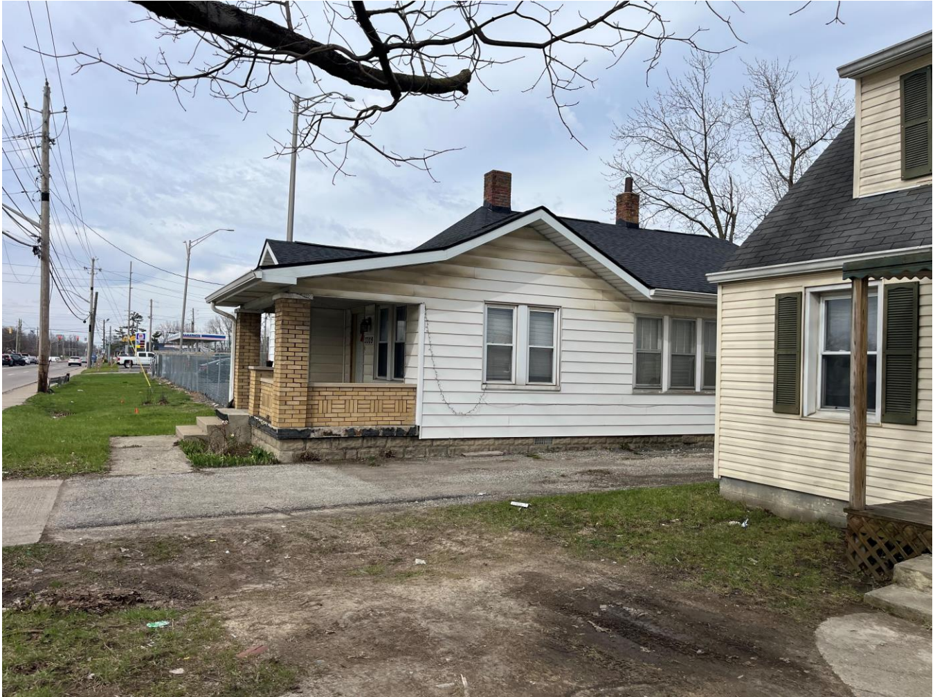
Photo 2: Single-family residence directly north of subject site.
