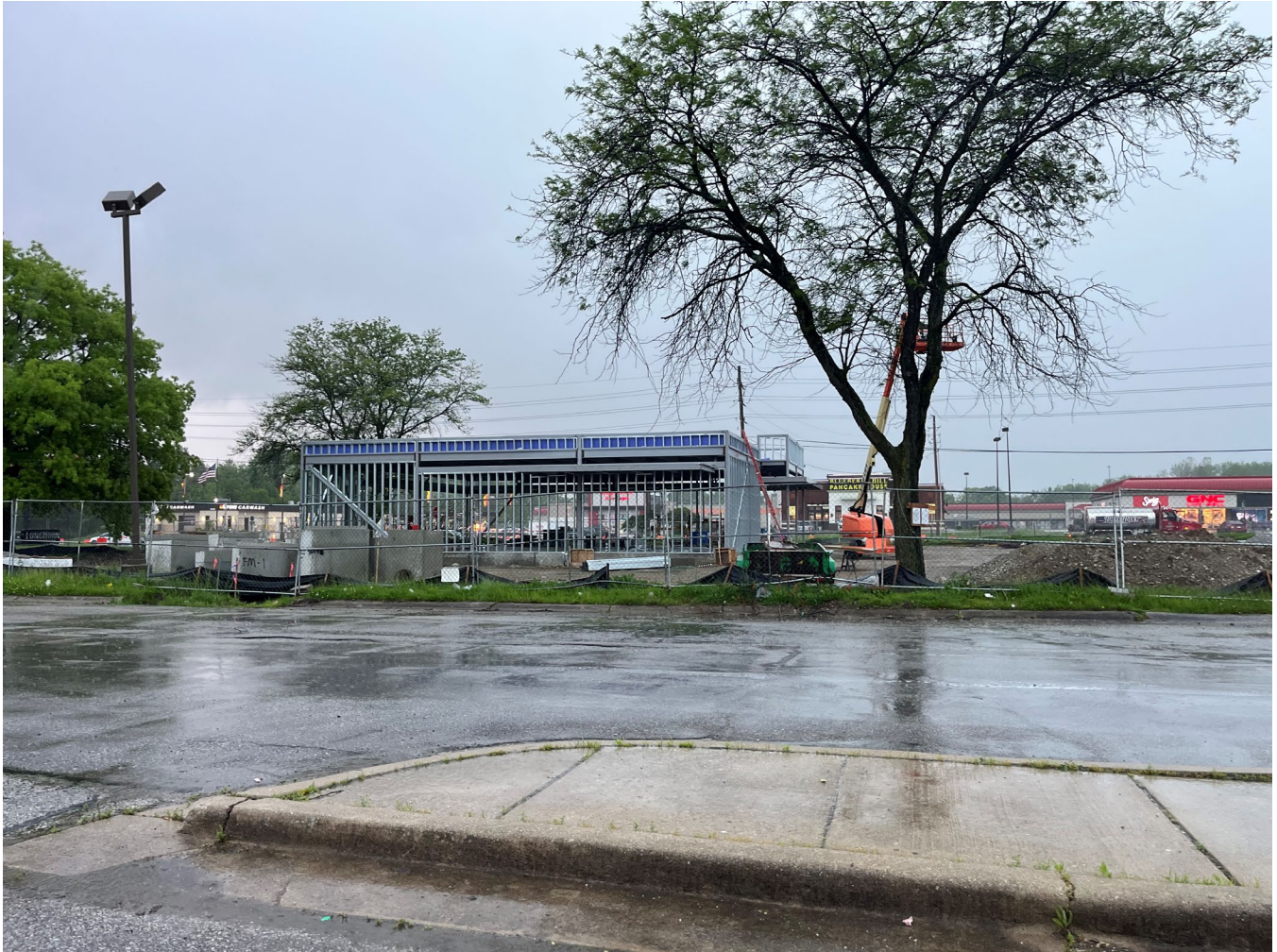
Photo 2: Framing of bank at subject site
