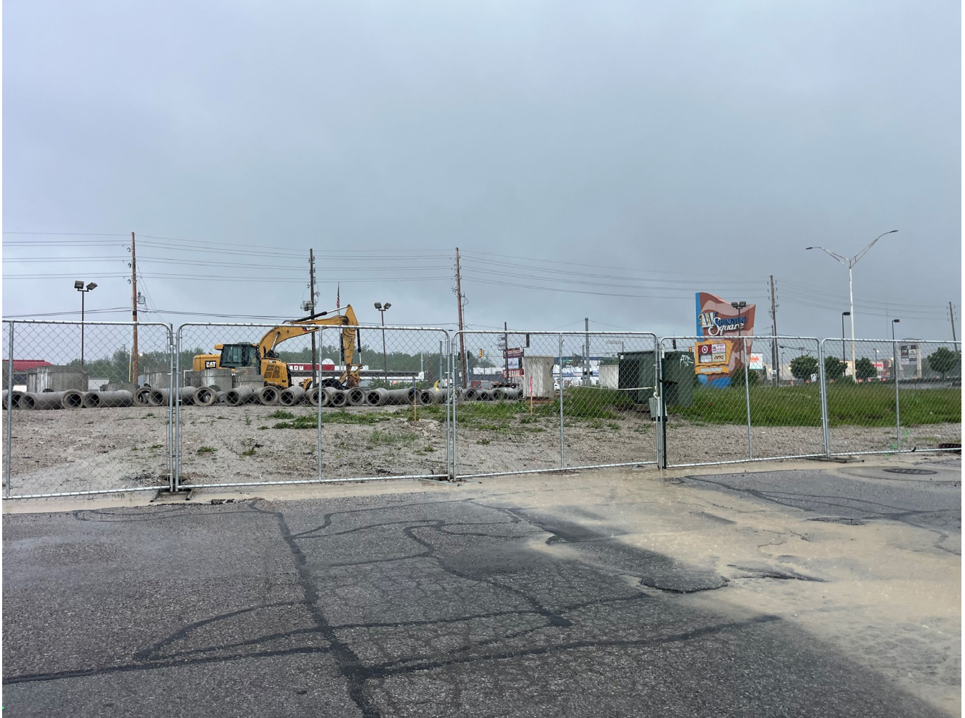
Photo 1: Subject site from mall parking lot
