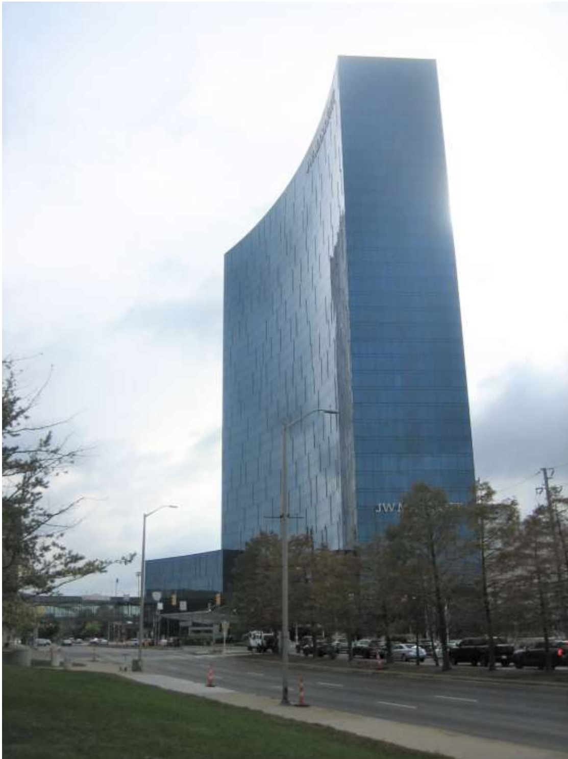
Subject site, looking south.
