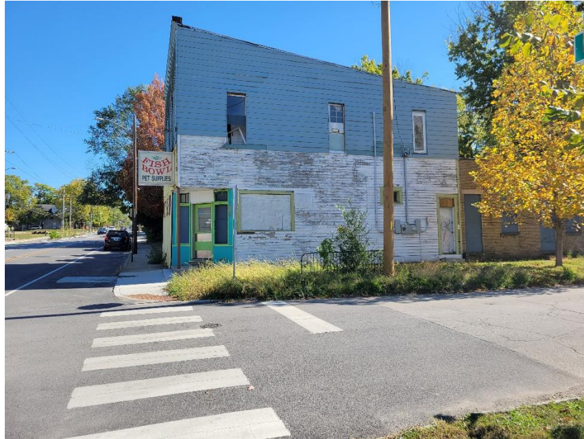
Photo 5: Adjacent Property to East
