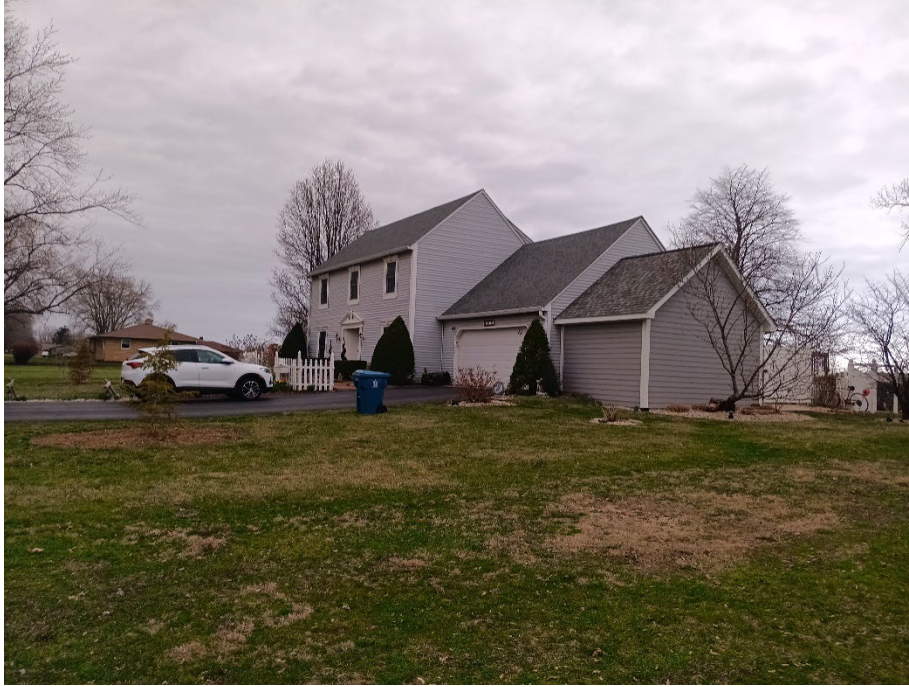
Exhibit 10: Home to the north of the subject site.
