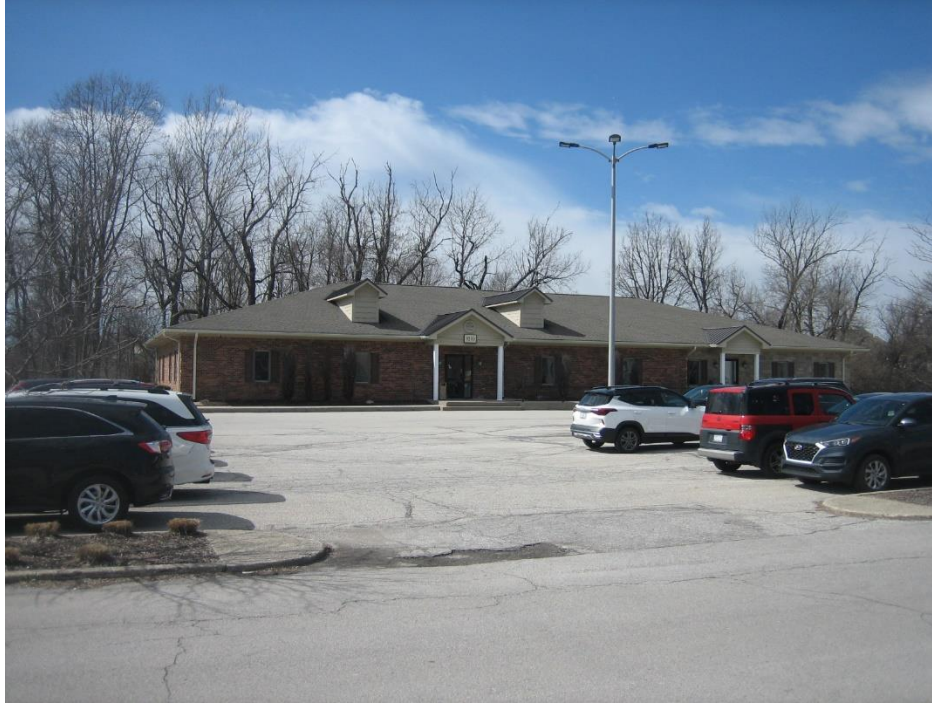
Subject site, looking west.
