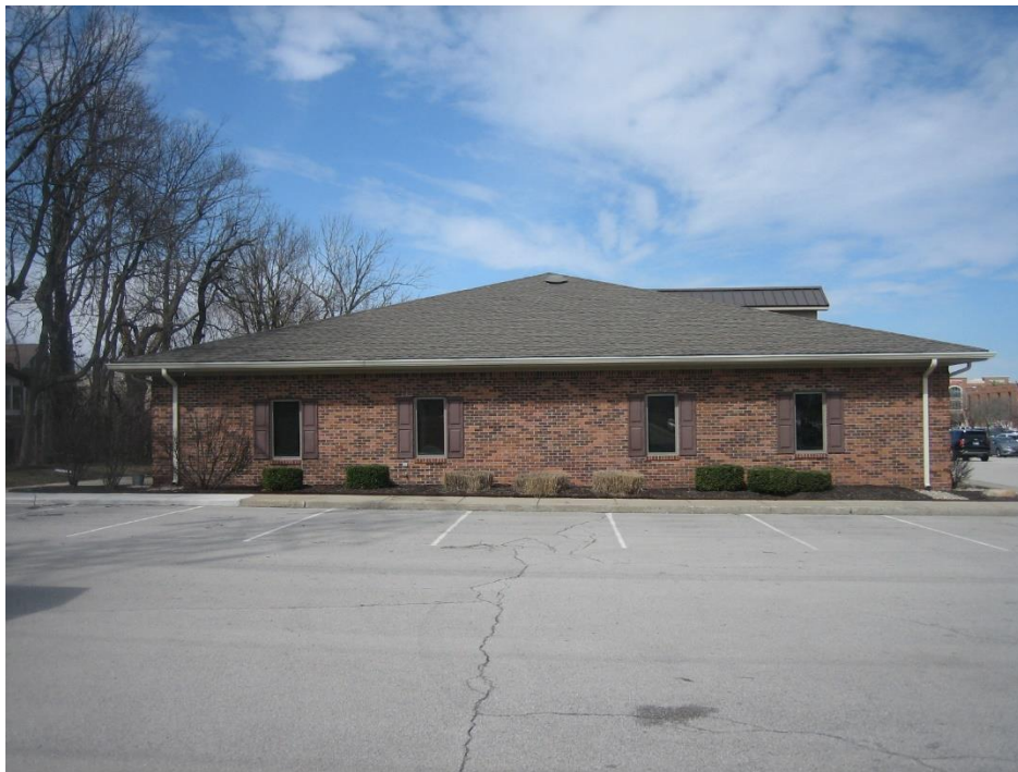
Subject site, looking north.
