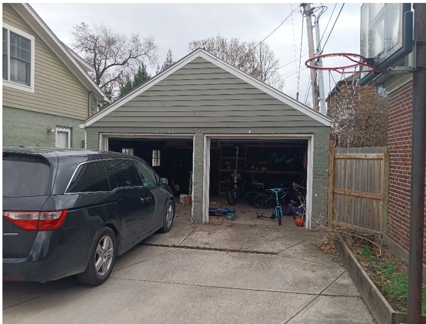
Exhibit 14: Existing Garage on the property.
