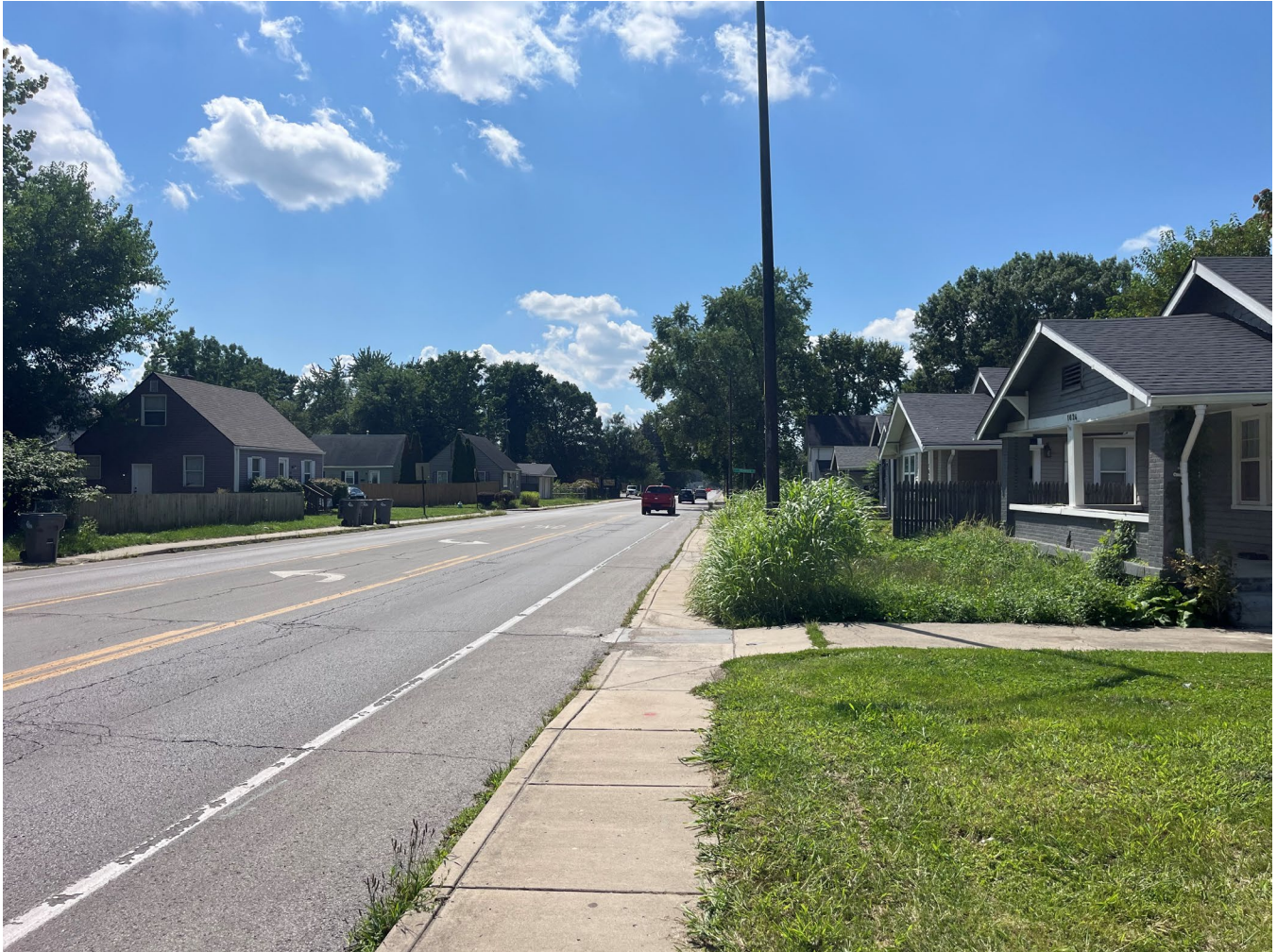
Photo 3: Looking west on 46 th Street
