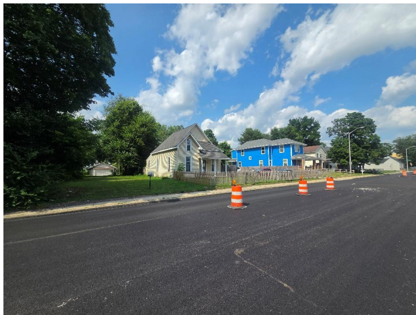
Photo 4: Adjacent Property to East
