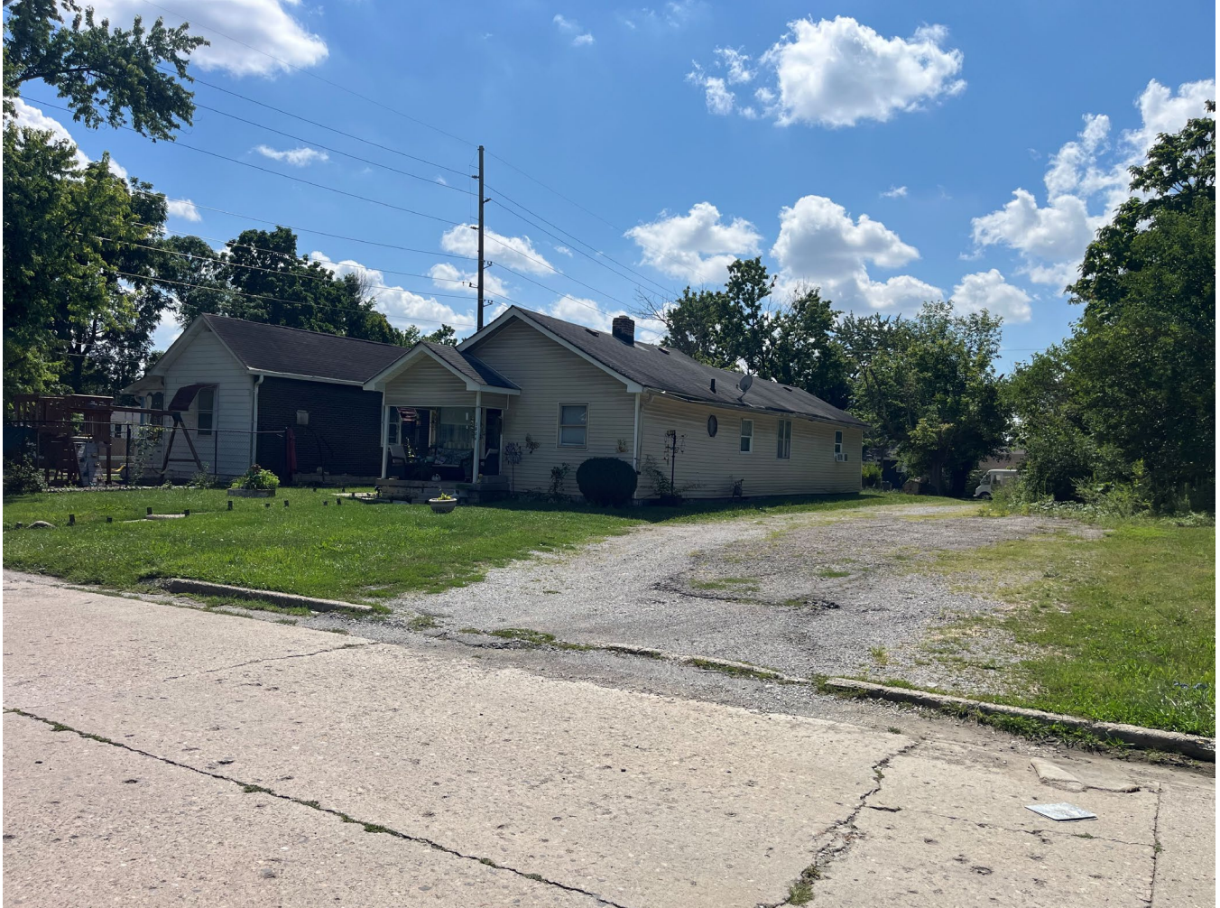
Photo 5: Looking across Gale Street
