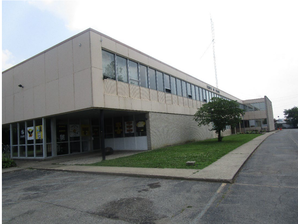
View looking southeast along existing building
