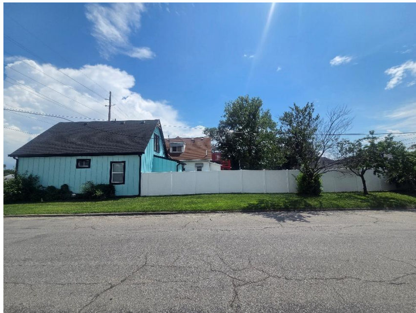
Photo 2: Subject Site Viewed from North
