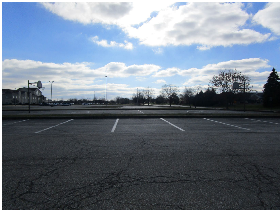
View of site looking south
